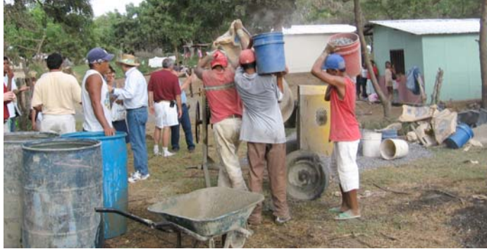
Homes being built by their future tenants at the fishing village of El Menco
